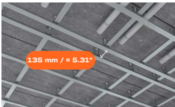
Installation width between profiles: 135 mm / ≈ 5.31"
